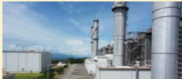
Ilijan Power Plant
