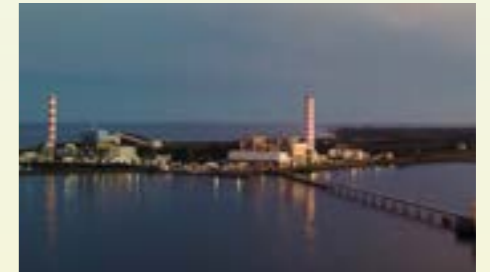
Masinloc Power Plant
