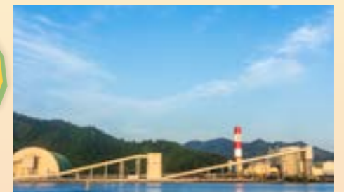
Malita Power Plant
