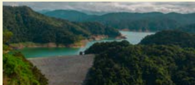
Angat Hydroelectric Power Plant
