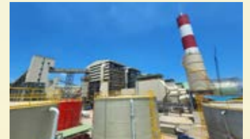
Mariveles Power Plant*
