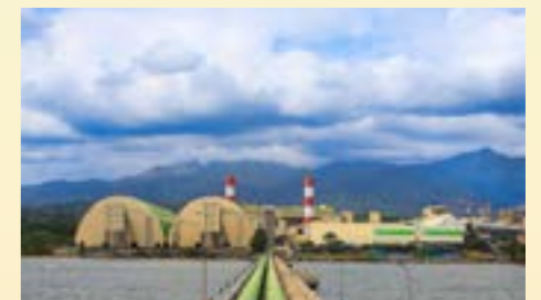
Limay Power Plant
